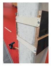
After the manufacturing, we mounted the tables to the concrete pillars in the B-building. This was not so easy, because the pillars have different sizes and angles, so that we had to adjust the sleeve a lot.
